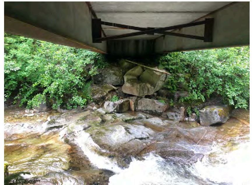
Left Bank Abutment when facing downstream
