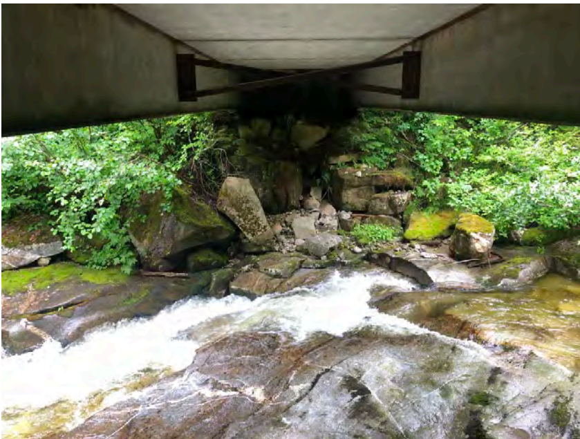
Right Bank Abutment when facing downstream
